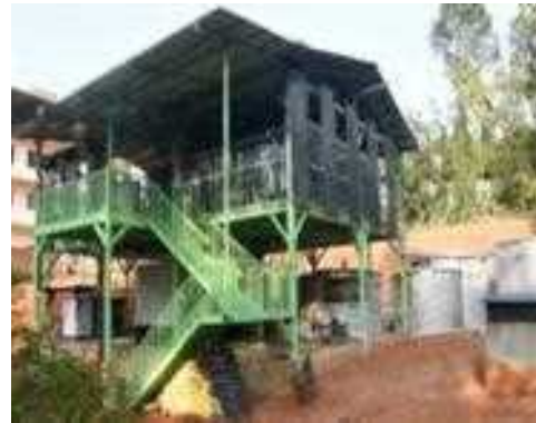
1 MLD STP at Kozhikode medical College
