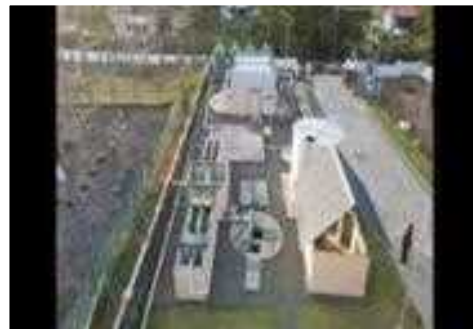
1 MLD CSTP at Padanappalam, Kannur
